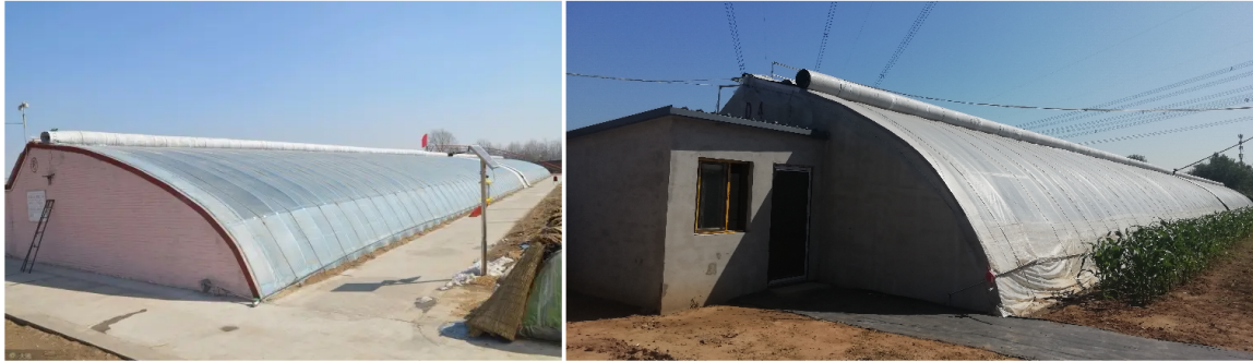
Fig. 1.2. Semi-fan shaped solar greenhouses.
