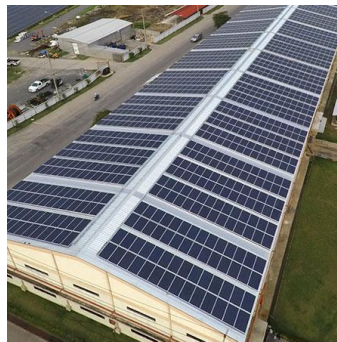
Figure 60. Panels over a roof
