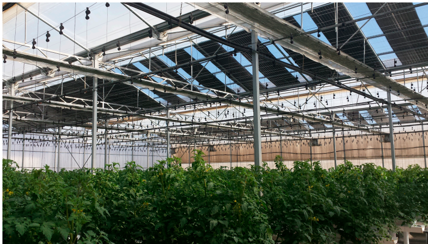
Figure 3. PV panels mounted on greenhouse roof. TECNOVA foundation experimental PV greenhouse (Almería).
