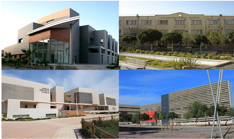
Figure 3 . Different buildings of the research and laboratory category.
