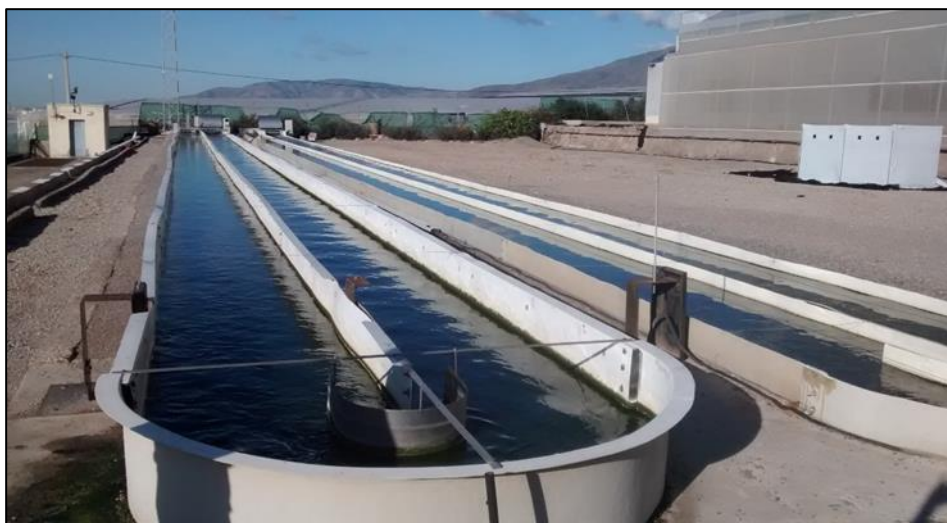
Figure 3.3. General view of the raceway reactors located at the "Las Palmerillas" experimental station in Almería (Spain) working in continuous mode from May 2016 to June 2018.
