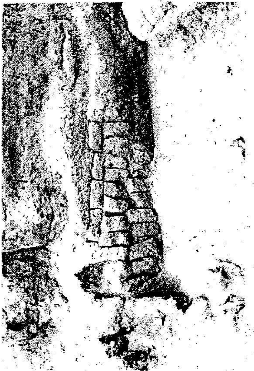
(Fig. 63) The Temenos wall shows how to strengthen, horizontally and vertically the layers (Al-Jumaili 1971: 84)
