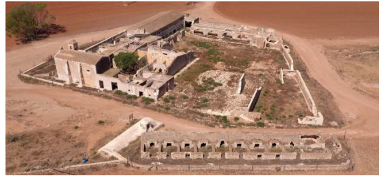
Fig. 3. Current state of ruin of the facilities of Cortijo del Fraile
