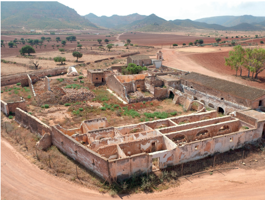
Figure 6. Perspective of the ensemble showing the semicircular arches in the stables of the Cortijo del Fraile.
