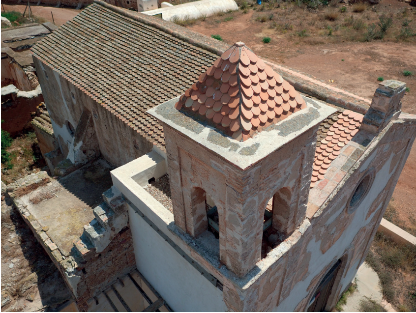
Figure 5. Detail of the bell tower.
