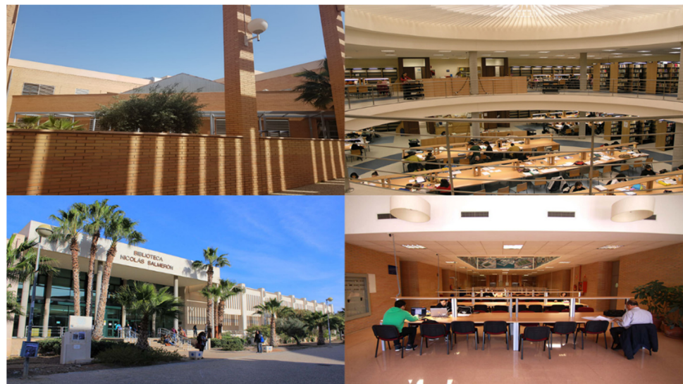
Figure 4. Different views of Library building.
