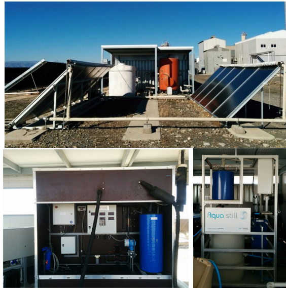
Figure 2: SMD pilot plant at PSA. From top to bottom and from left to right: solar field, Solar Spring module, and Aquastill module.
