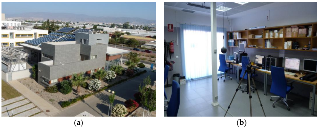
Figure 2. Center for solar energy research (CIESOL) building (a) and the laboratory under study (b).
