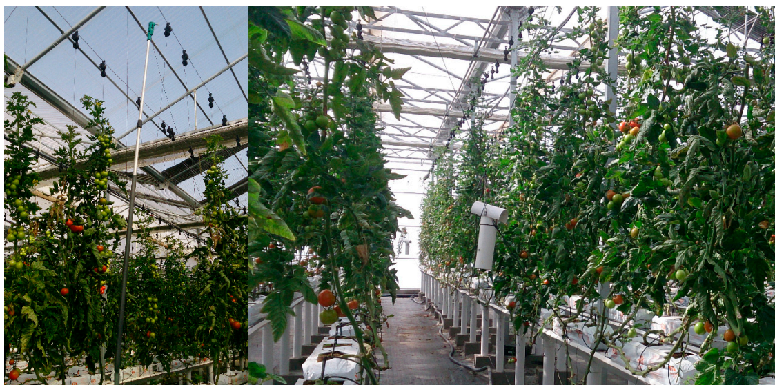
Figure 6. Detail of installation of radiation (left) and temperature (right) sensors.
