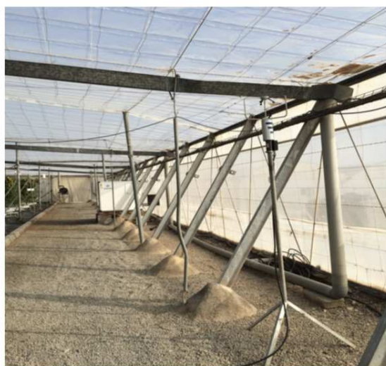
(a) Lateral windows in greenhouse situated in Las Palmerillas
