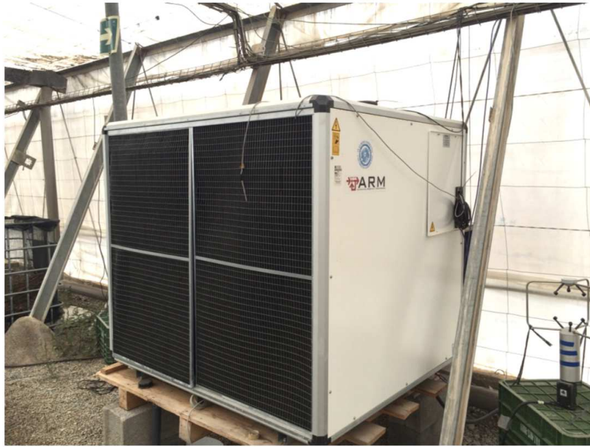
Figure 2.2: Deshumidificator located inside greenhouse in Las Palmerillas. Image taken from [2]
