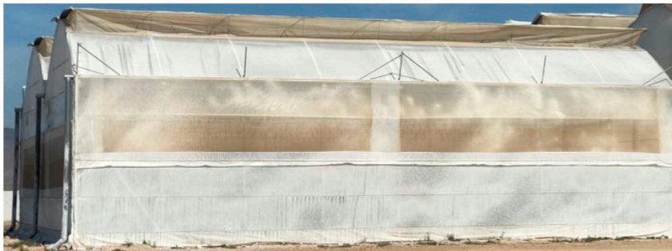
Figure 1. Greenhouse with fan-pad system.
