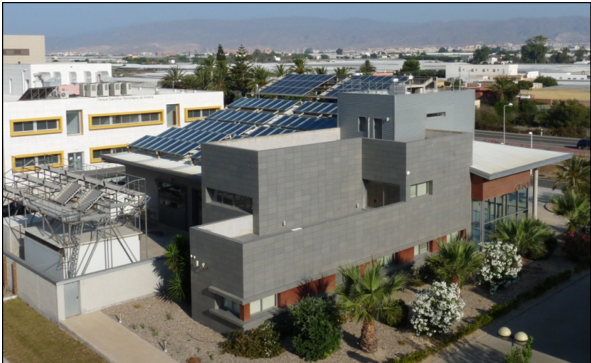
Figure 3.1. Backside picture of the CIESOL building where the photovoltaic field and the field of solar collectors are visible in the rooftop
