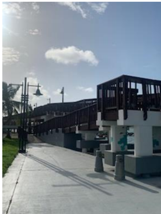
Photo 16-Boardwalk with view towards the San Juan Bay, Cataño, Puerto Rico. Source: Own creation.
