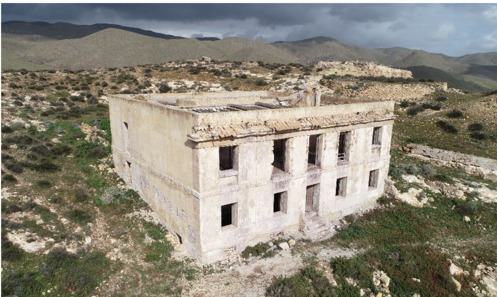
Fig. 4 View of the reservoir administration building
