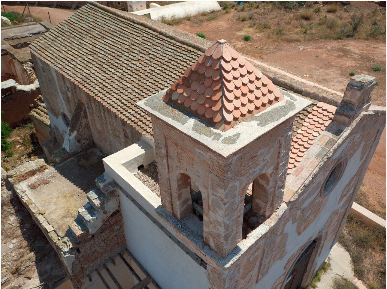
Figure 5. Detail of the bell tower.
