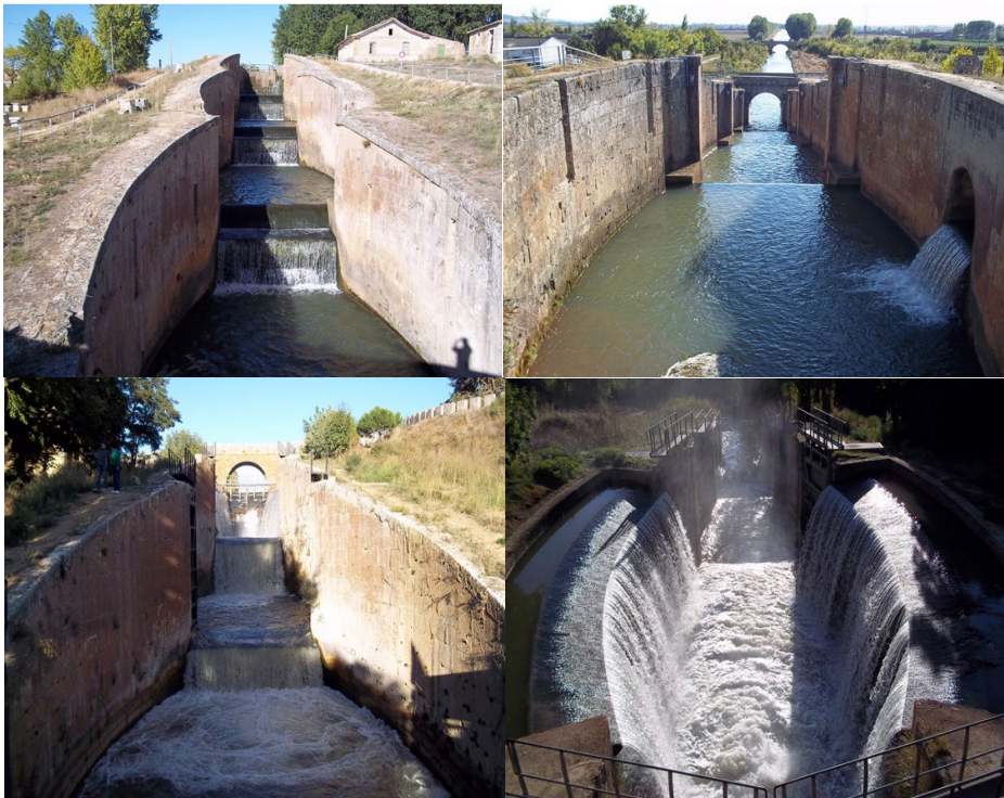
Figure 3: Locks along the Canal de Castilla
