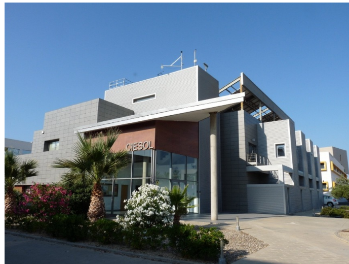
Figure 6. The CIESOL building.
