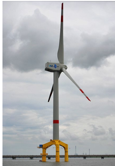
Figure 7. Bard 5 MW wind turbine over a tripile foundation.
