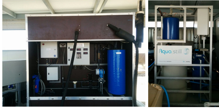
Figure 7: Commercial MD modules at PSA. From left to right: Solar Spring and Aquastill modules.
