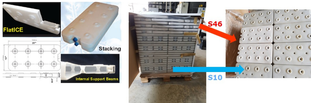
Figure 12. FlatICE containers installed in the CIESOL building (based on [34]).
