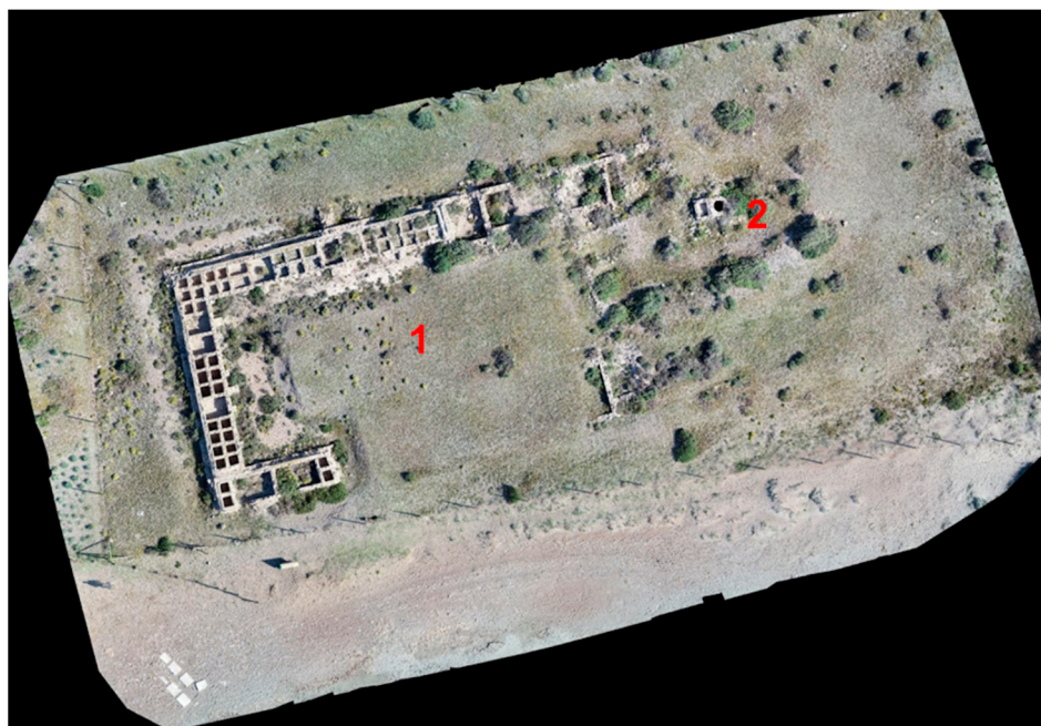
Figure 3. Orthophotography zenithally view of the site. 1: central courtyard of the building; 2: location of the hydraulic supply structures.
