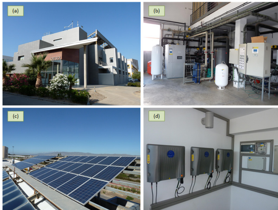
Figure 1. The Solar Energy Research Center (CIESOL or Centro de Investigación en Energía SOLar in Spanish) building: (a) exterior of the CIESOL building; (b) solar cooling installation; (c) photovoltaic (PV) power plant: PV panels; and (d) PV power plant: PV inverters.
