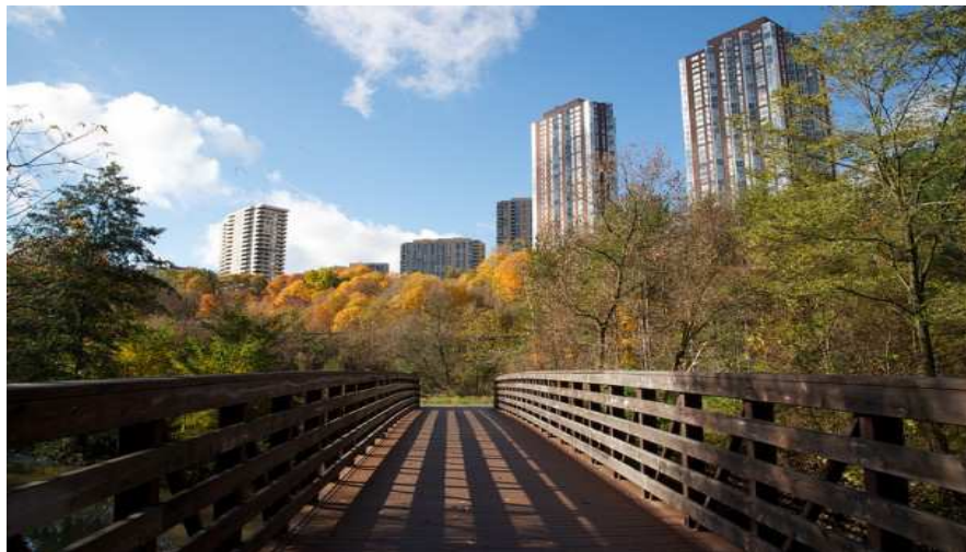
Fig. XIV. [Bridge over Don River]
