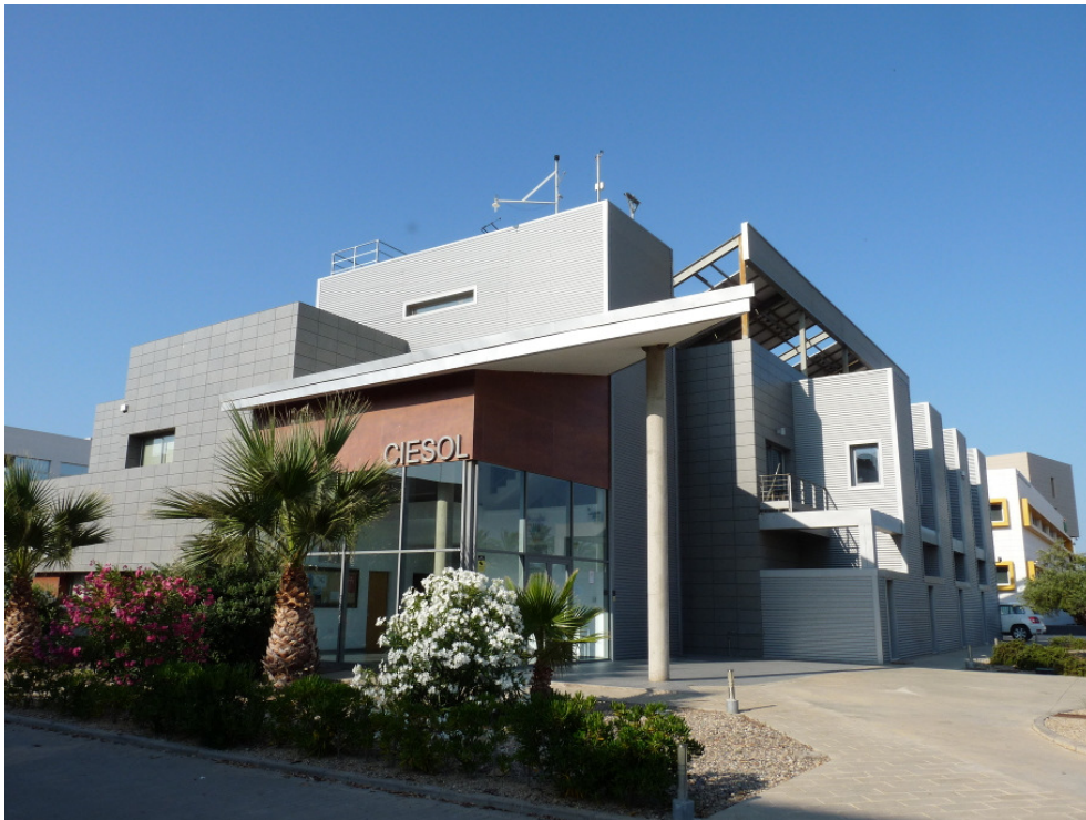
Figure 1. The CIESOL building.
