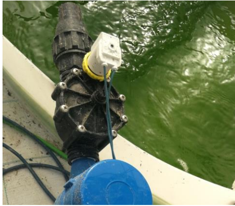
Figura 2.29 Electroválvula 2/2 8301BPNC24AC Euro-Rain.
