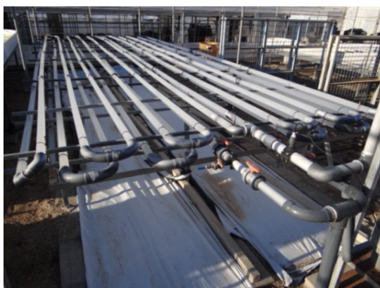
Figure 1. View of the experimental tubular photobioreactor.
